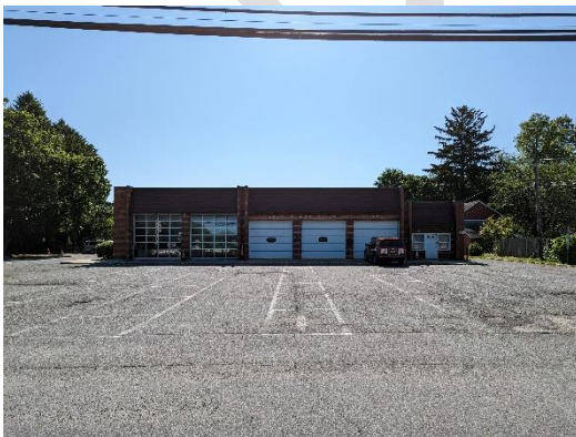
Image 15: Volunteer Fire House
