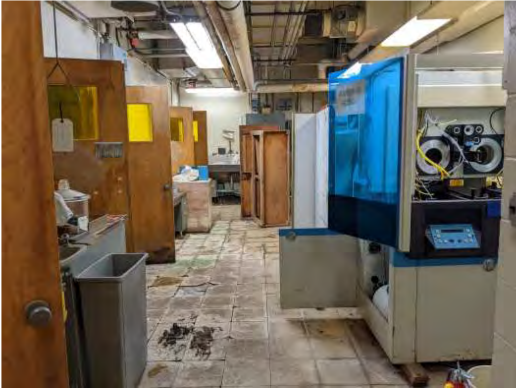
Photograph 24: Evidence of vacant lab space (Building 4)
