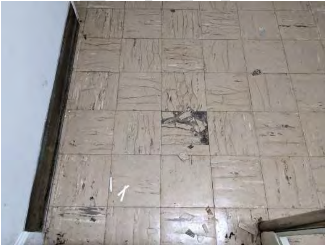
Photograph 8: Asbestos tiles
