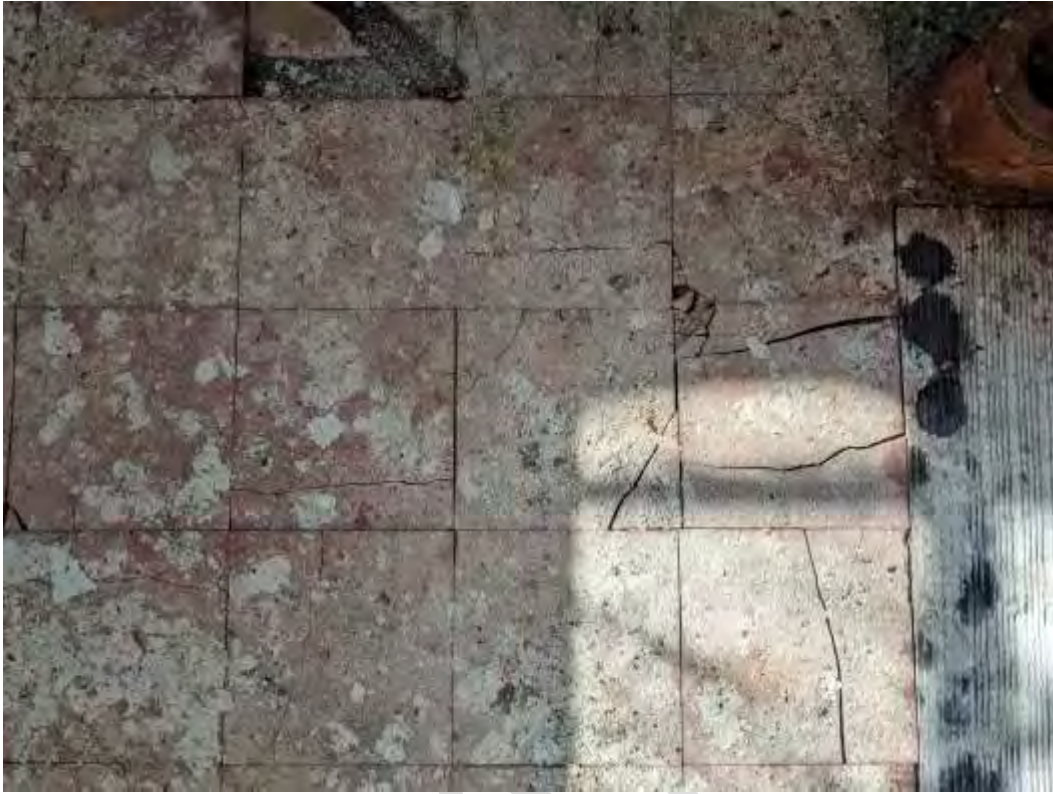
Photograph 9: Asbestos tiles
