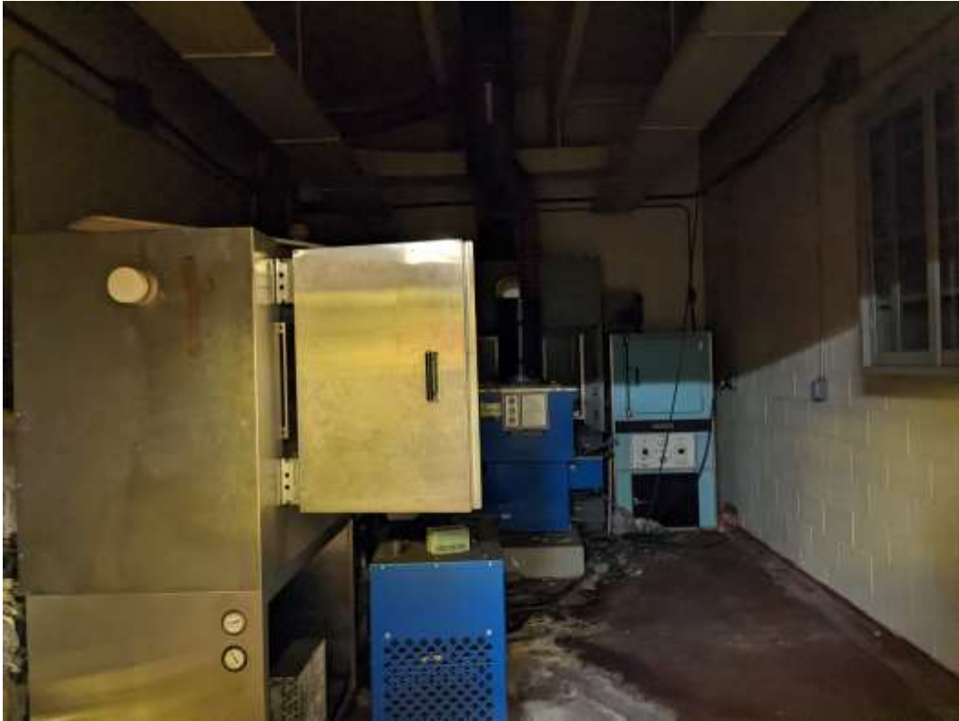
Photograph 26: Evidence of vacant lab space (Building 4)
