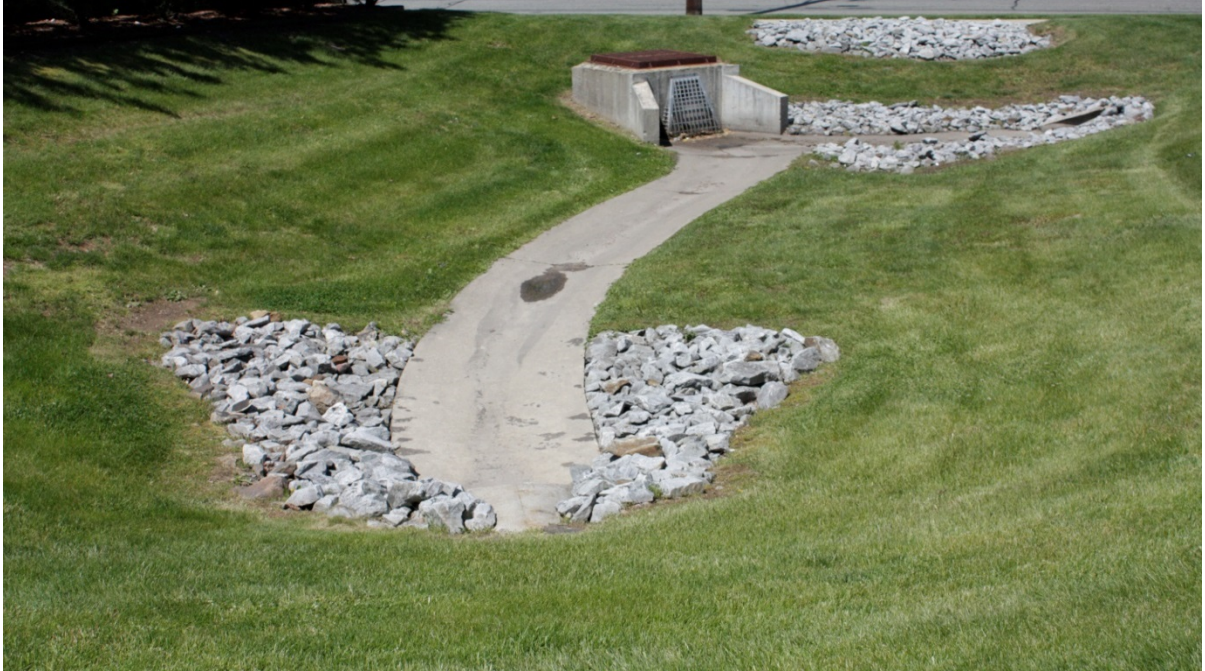
A well maintained detention basin
